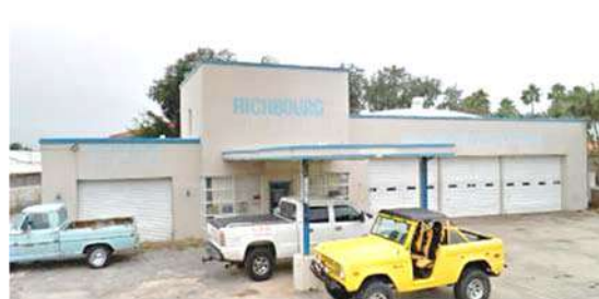
Buildings designed to facilitate automobile access to bays (building far from the sidewalk, one story, repair bay doors, canopy)
