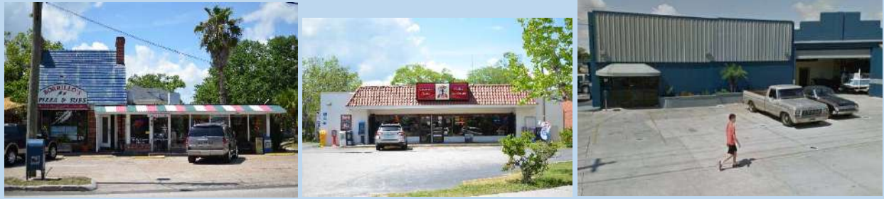
Figure 25: Examples of Existing Non-Conforming Parking Facilities
