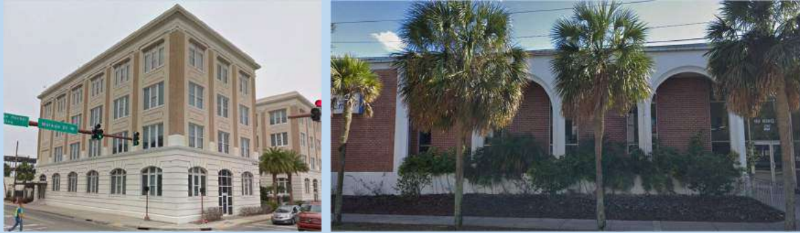
Allowed – Left: Brick counts as one of the three colors; Window trims and door provide accent colors
