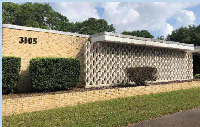
Figure 2. Existing Structures at Jacksonville University. Note use of geometric screen walls, yellow brick, and horizontal lines.
