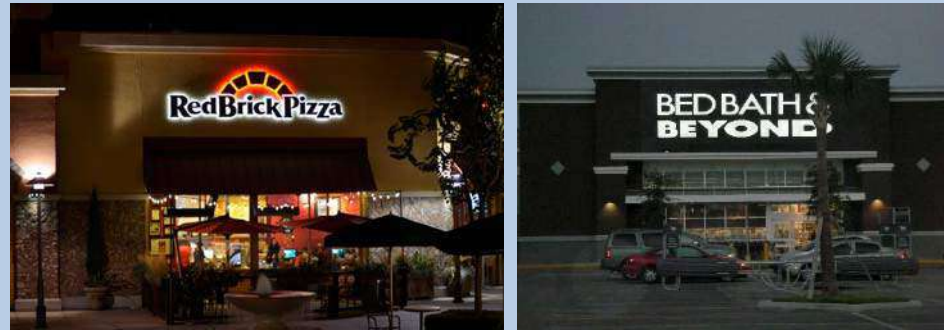
Figure 39. Prohibited Sign Illumination
