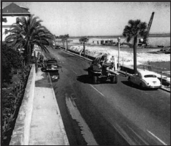
Prior to road widening, 1957-9
