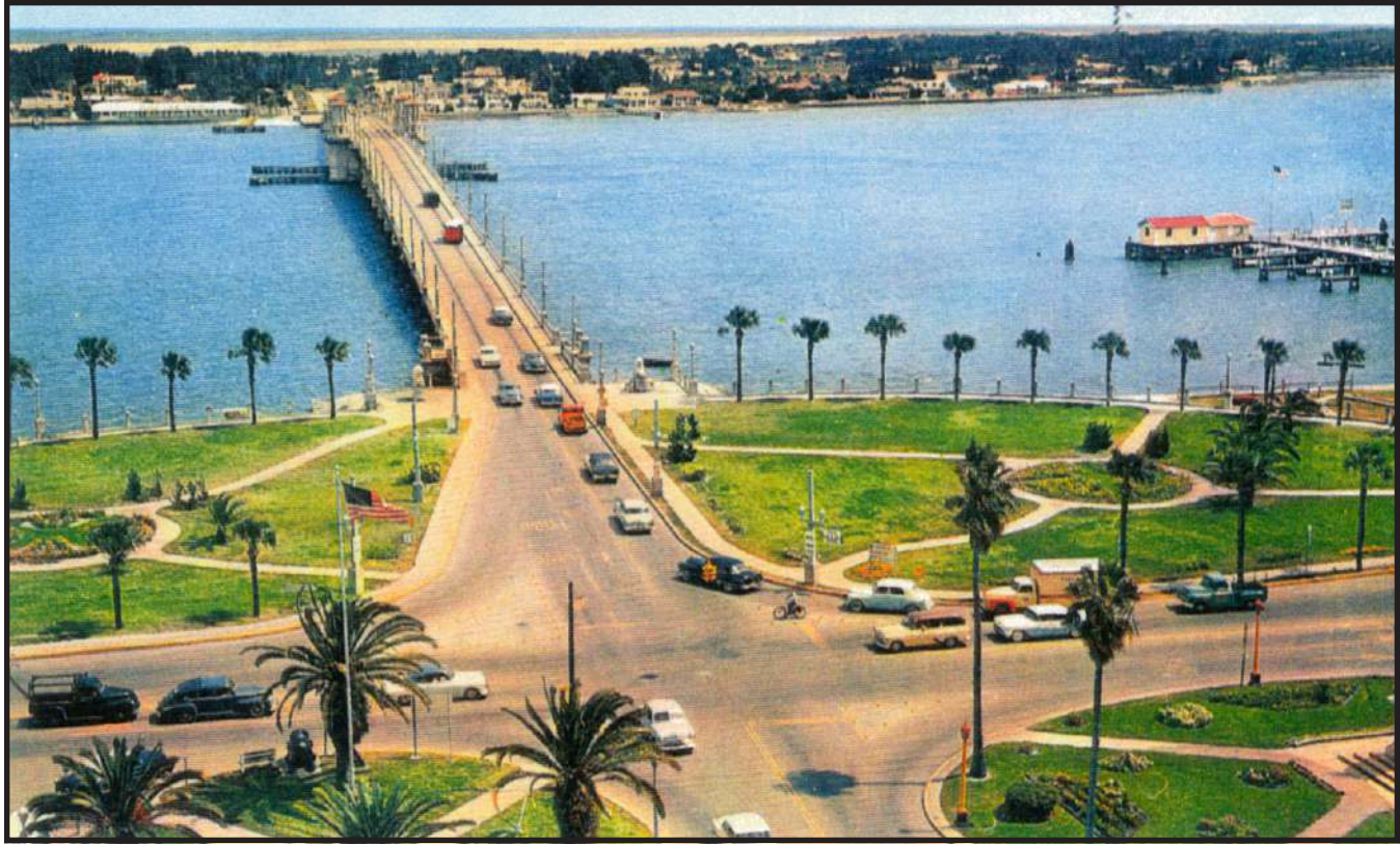
Color postcard of Avenida Menedez prior to road widening, early 1950's
