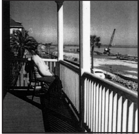
View east toward construction, 1957-9
