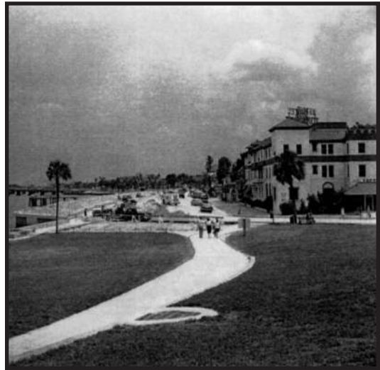
View south toward construction, 1957-9
