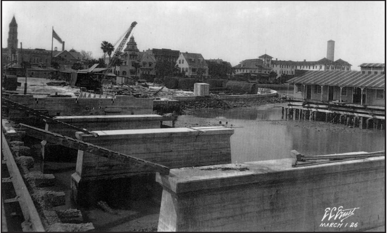
West abutment, March 1926
