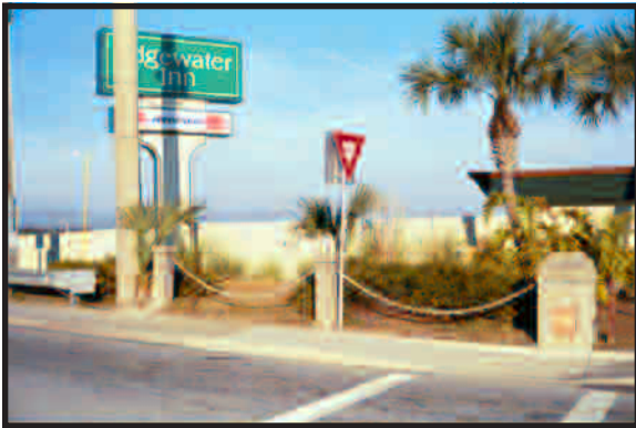
Railing system in front of Edgewater Inn
