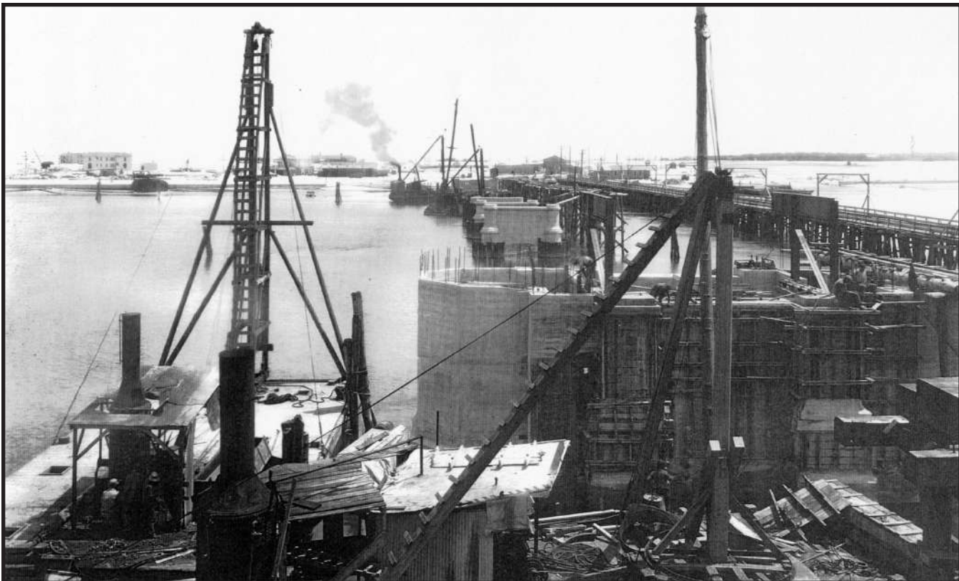
Construction of west abutment, September 1926
