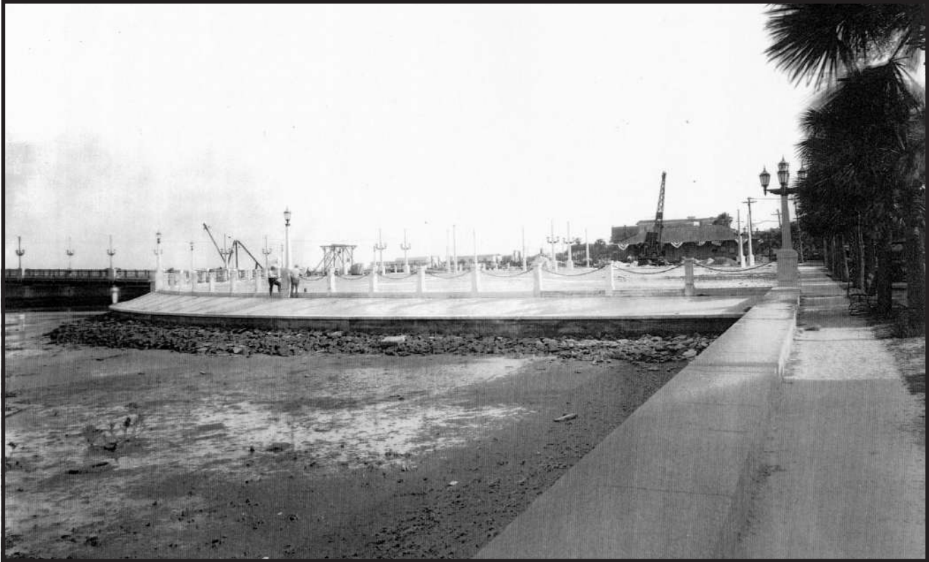
North end of west park approach, undated
