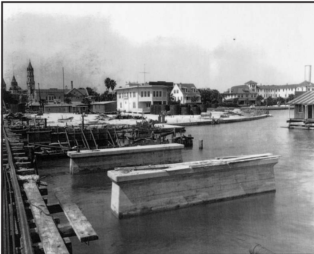
Bridge forming at west approach - northwest view, 1925
