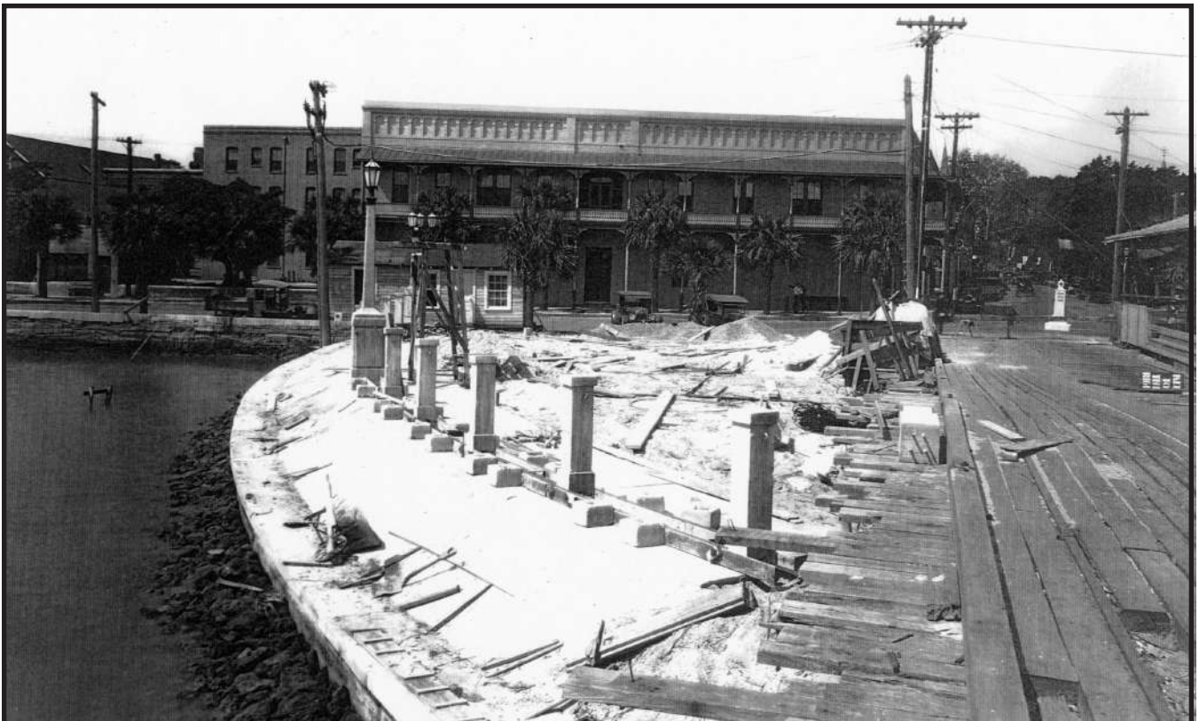
Precast concrete post and chain construction at west plaza, April 1926
