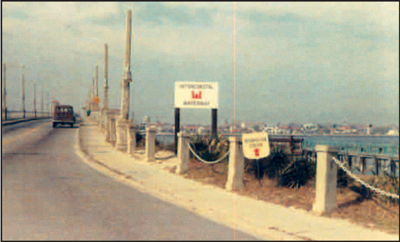
View west over bridge with original lamp posts, 1967
