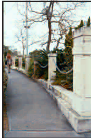
Railing system adjacent to miniature golf course
