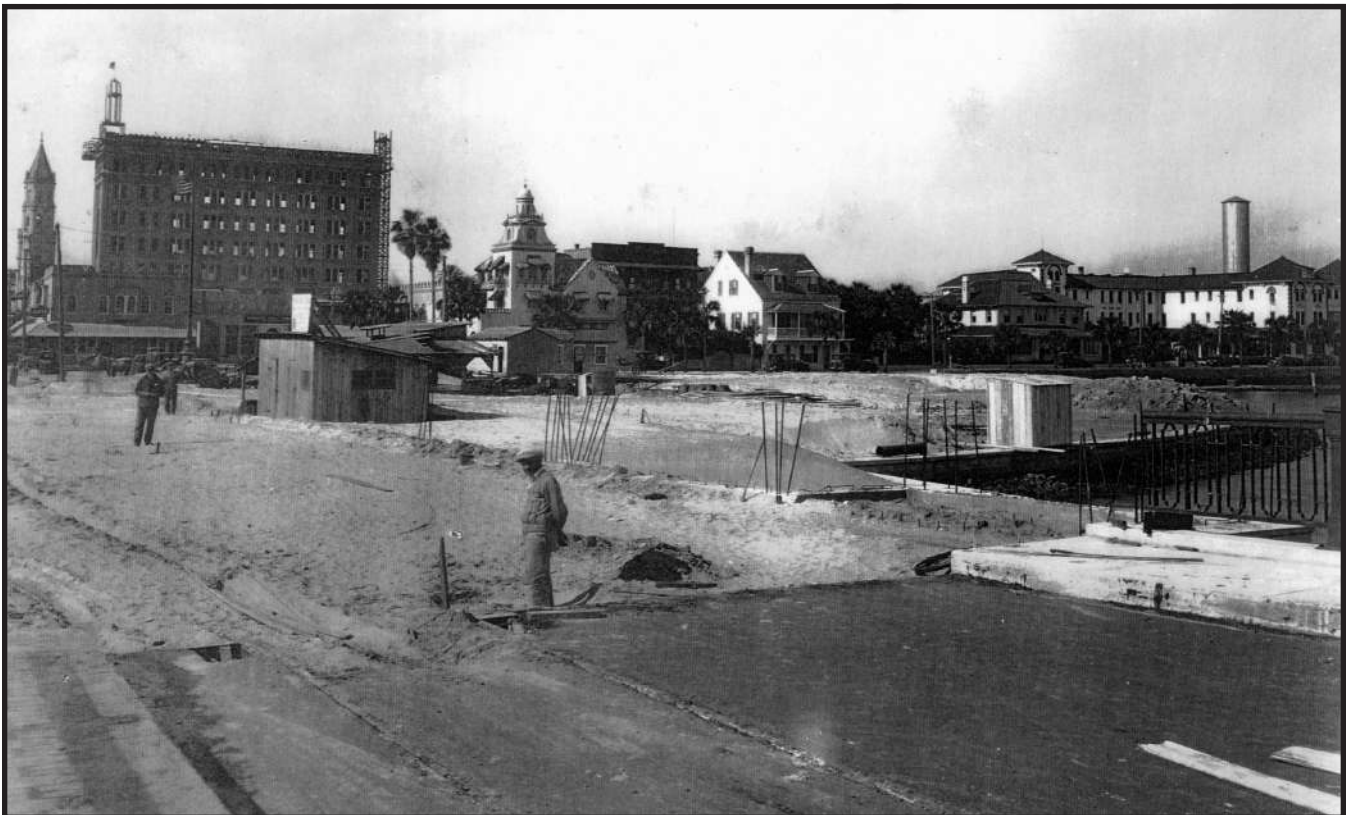
Construction of west bridge approach, January 1927
