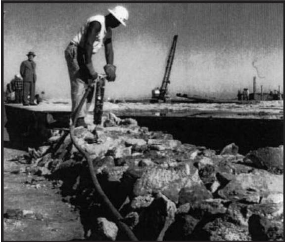
Breaking up of old seawall, 1957-9
