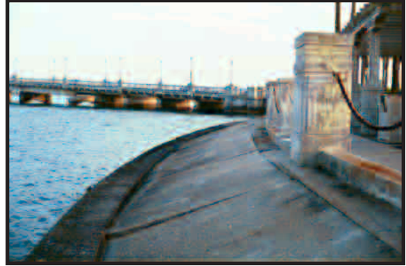
North portion of west park bulkhead
