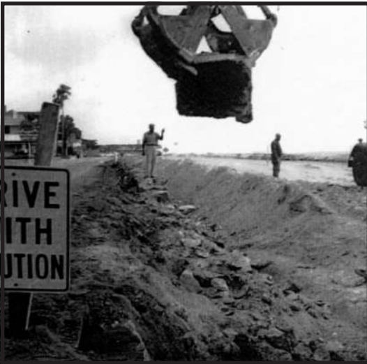
Removing old seawall, 1957-9
