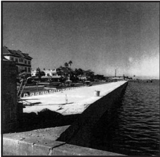
End of new seawall, 1957-9
