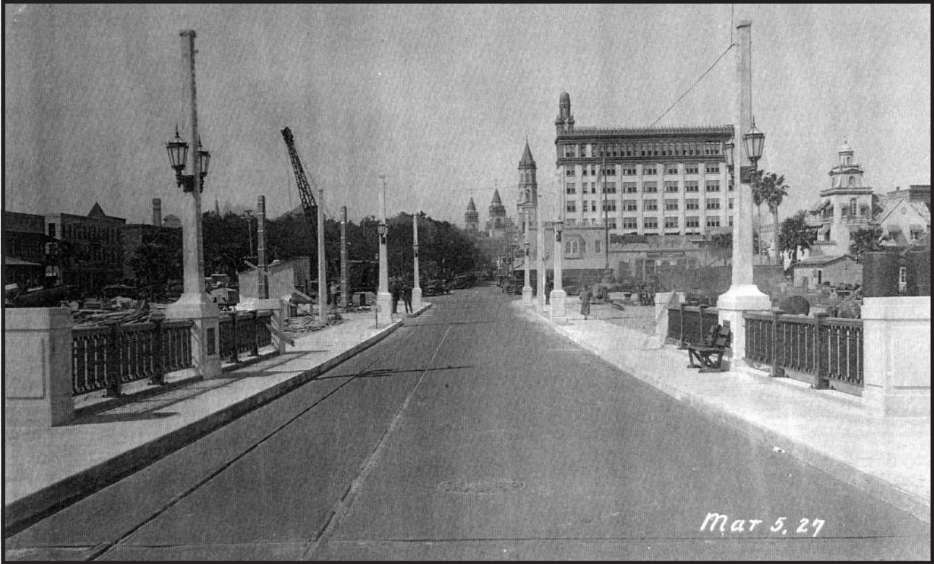
Completed bridge, facing downtown St. Augustine, March, 1927
