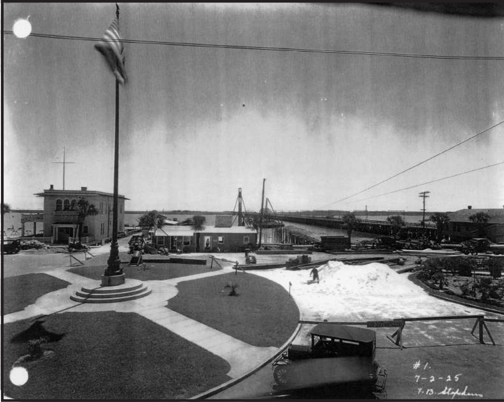
View over Anderson Circle of bridge under construction, July 1925
