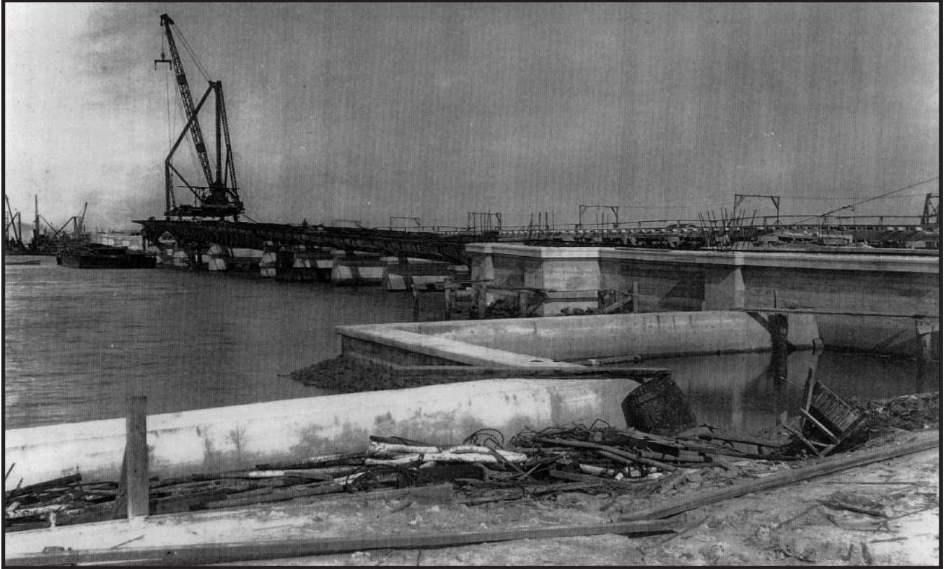
Bridge deck construction facing east, July 1926
