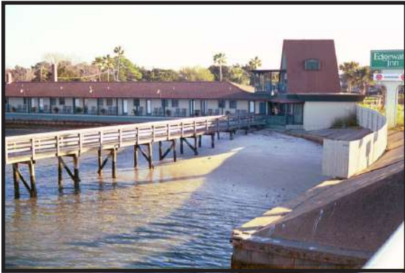
Pier and bulkhead at Edgewater Inn
