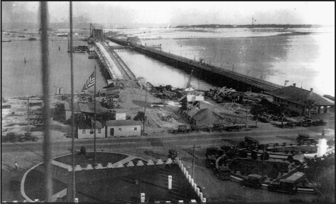
1927 view of bridge construction behind Ponce de Leon Circle
