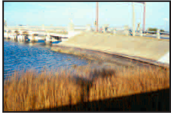
South portion of bulkhead at east park approach
