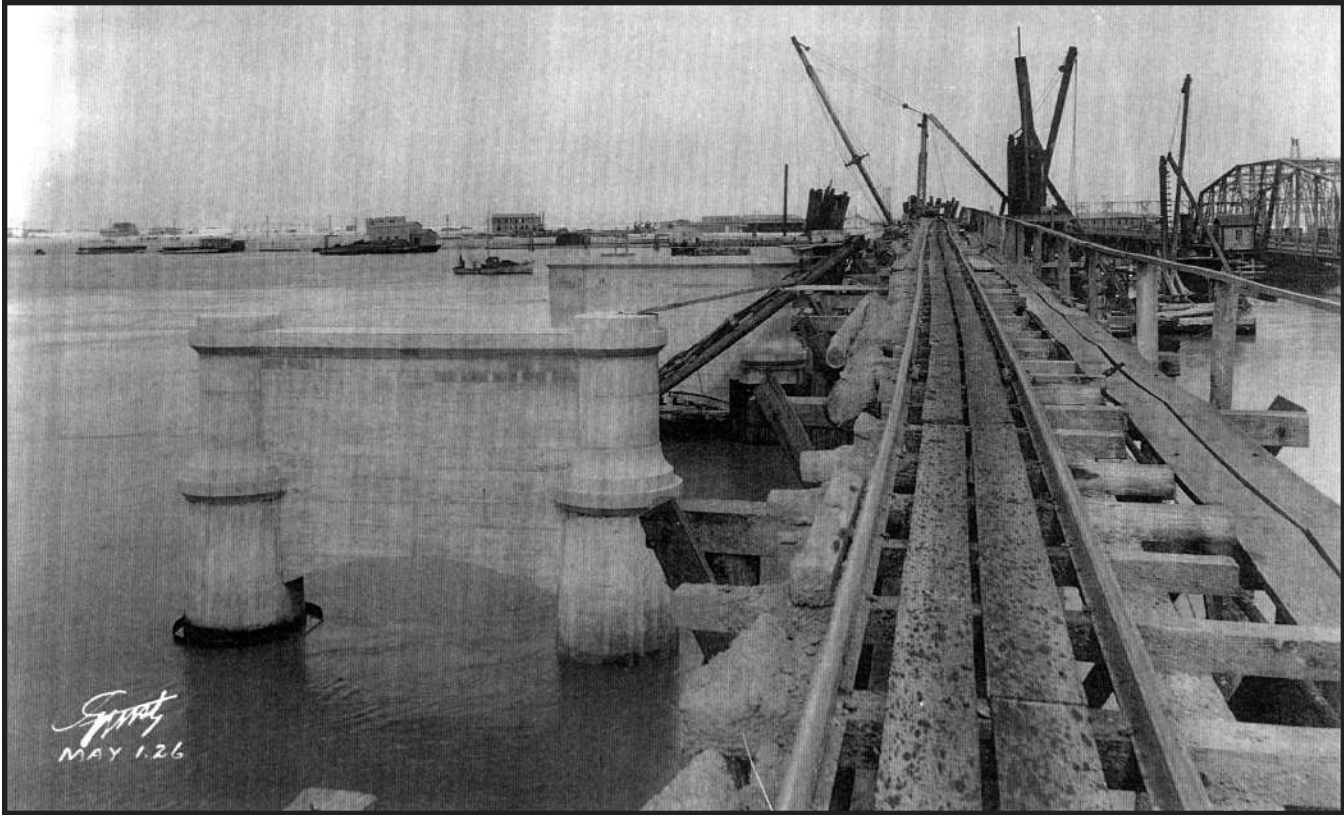
Forming of concrete piers - view east toward Davis Shores, May 1926
