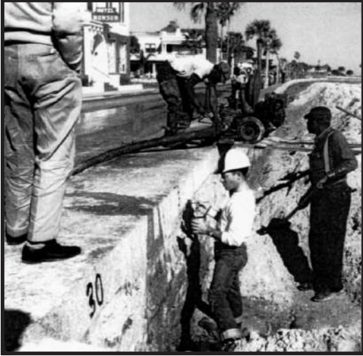
Workers on old seawall, 1957-9
