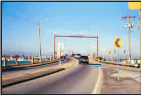
Concrete median at east park approach
