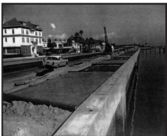
Paving the new esplanade, 1957-9
