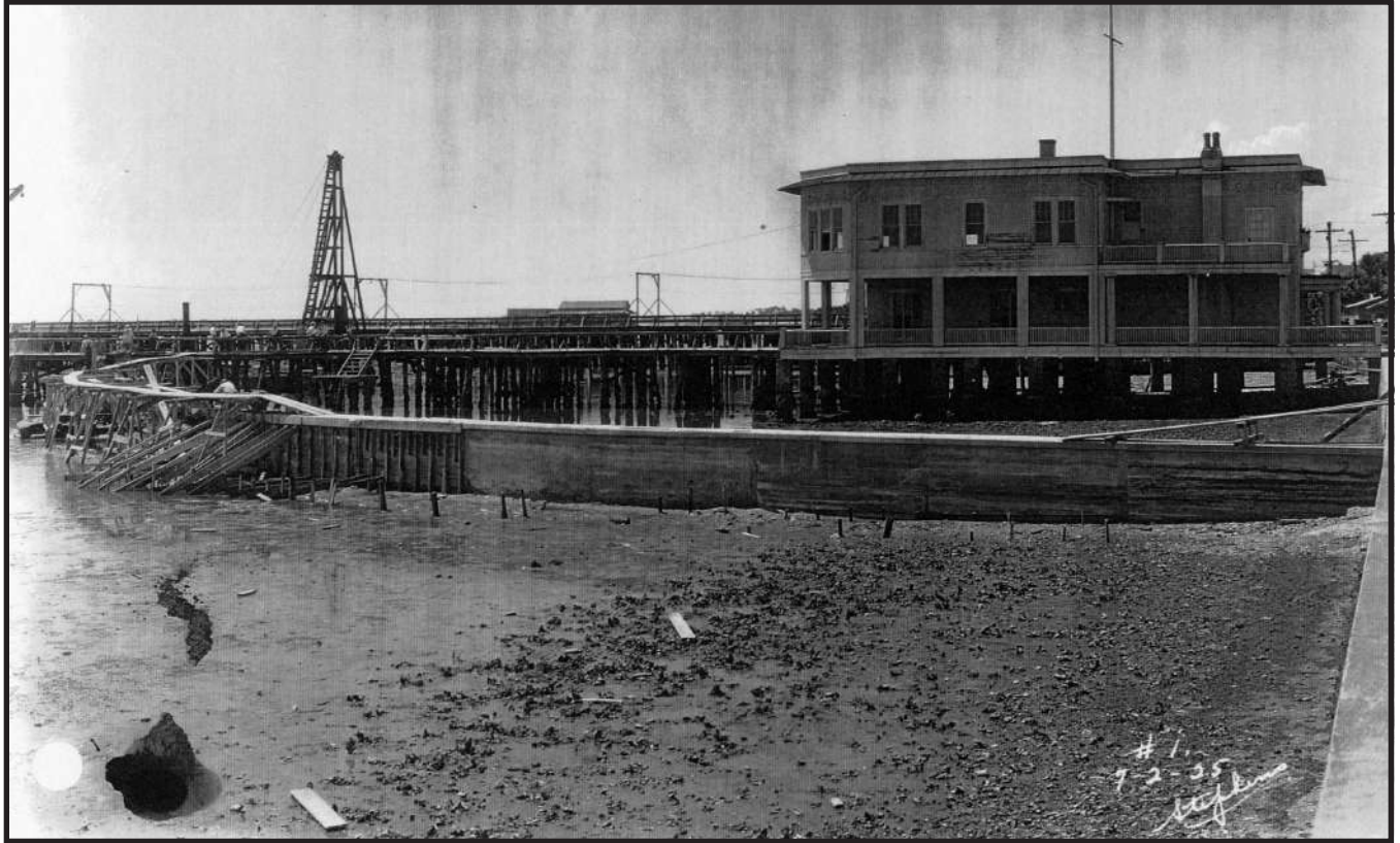
Forming of bulkhead at plaza of west park approach, July 1925
