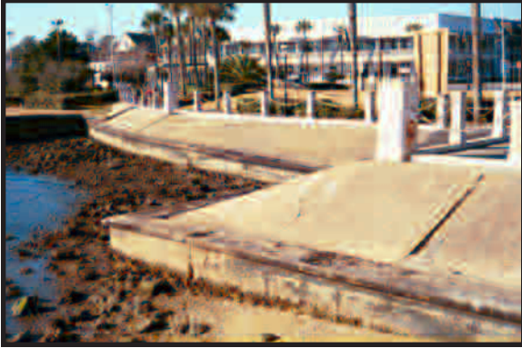
South portion of west park bulkhead
