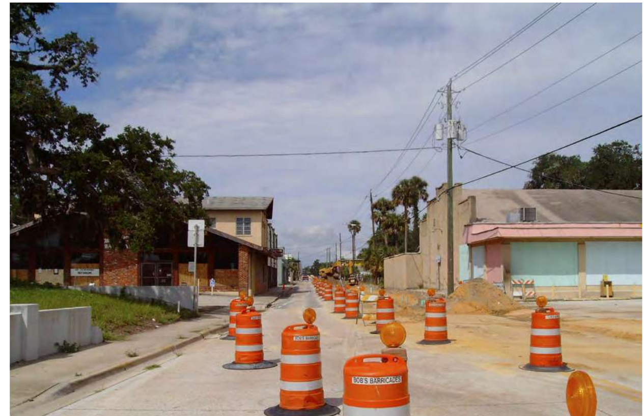
BEFORE Looking west on King Street, towards West Augustine.
