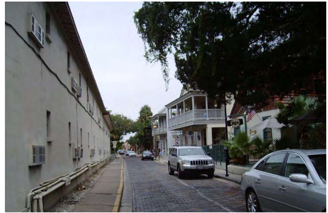
BEFORE Looking south, adjacent to the Monterey Inn hotel.
