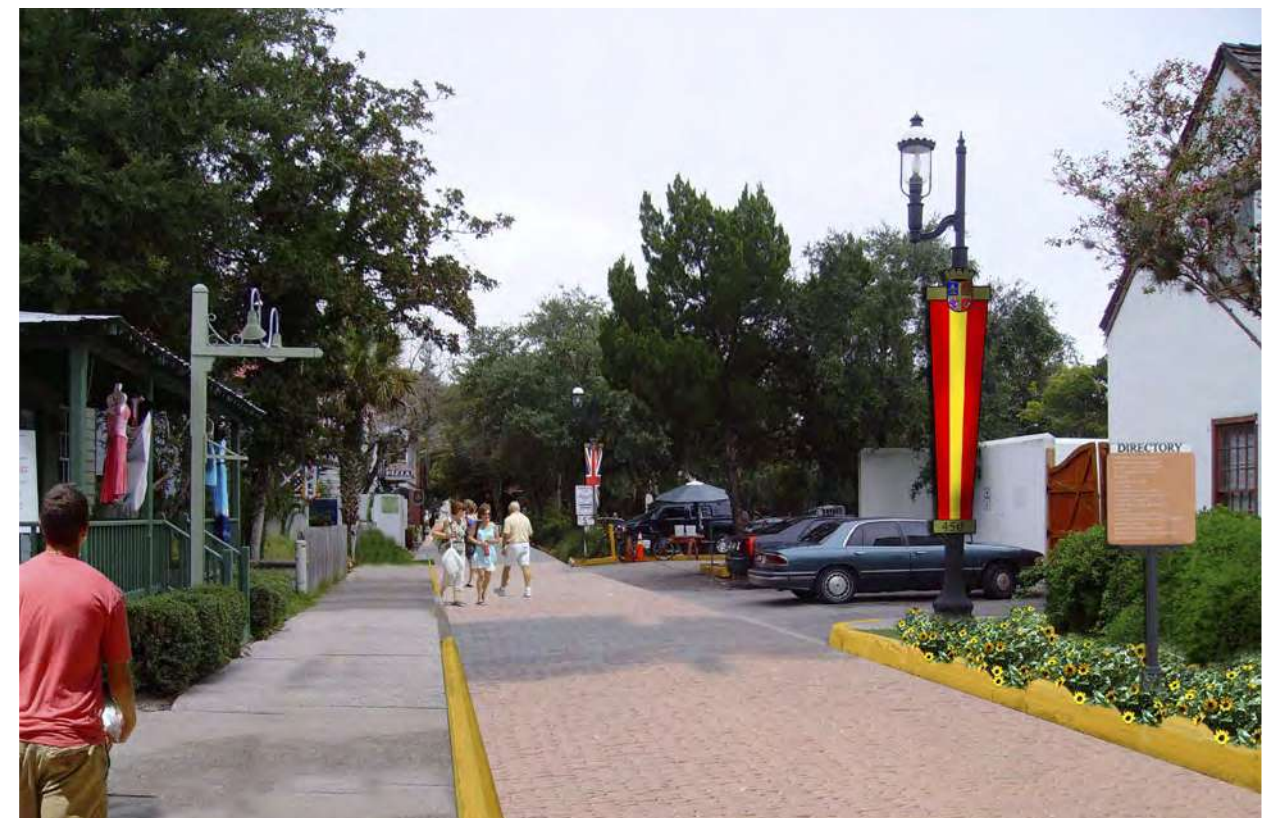
AFTER The asphalt has been replaced with historic bricks, which helps to integrate Spanish Street into the fabric of downtown. Converting the street to one-way traffic allows an expanded sidewalk to be installed.
