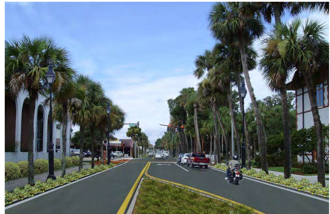
AFTER A raised median, low maintenance plantings, new lighting, new asphalt, and underground utilities transforms this important corridor.
